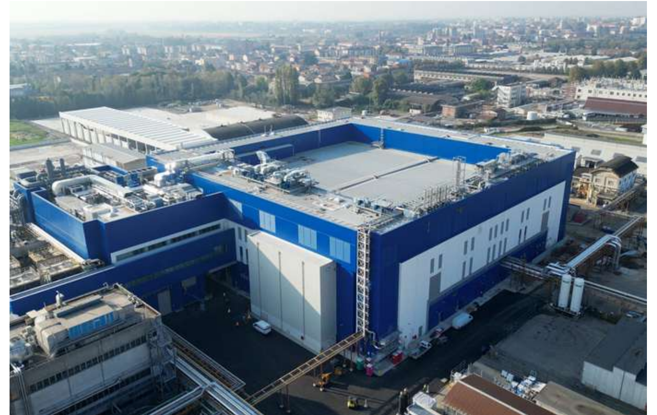
Pictured: Memc's new plant, Novara
